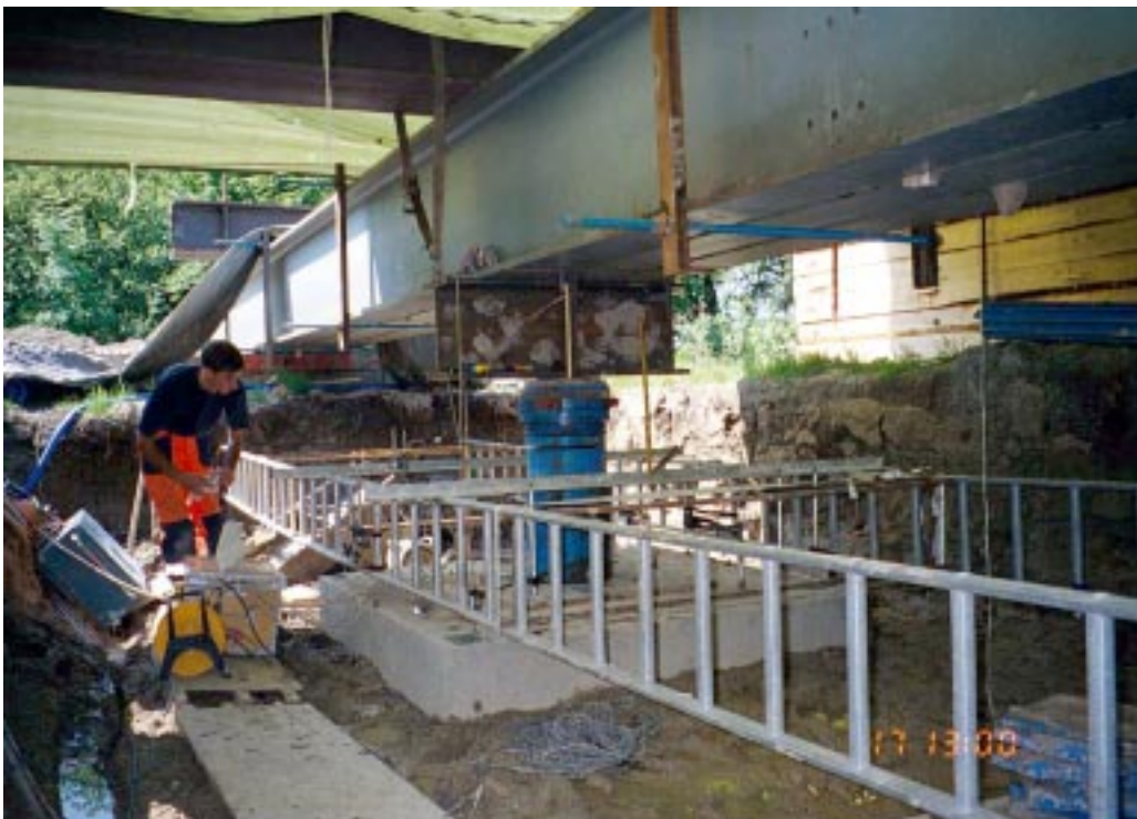
Fig. 83. Installation of the measuring system.
