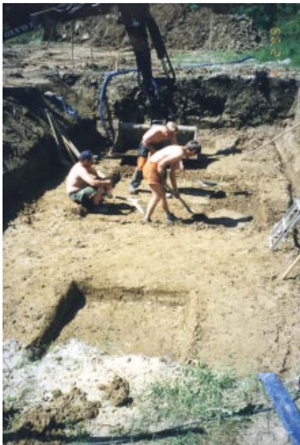
Fig. 81. Excavation for the plates at Tornhill.
